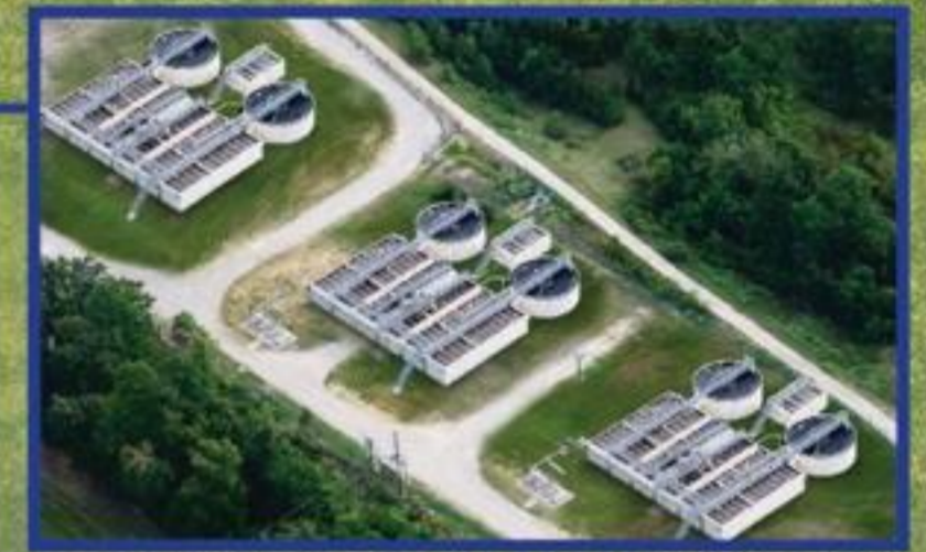
WASTE WATER TREATMENT PLANT
