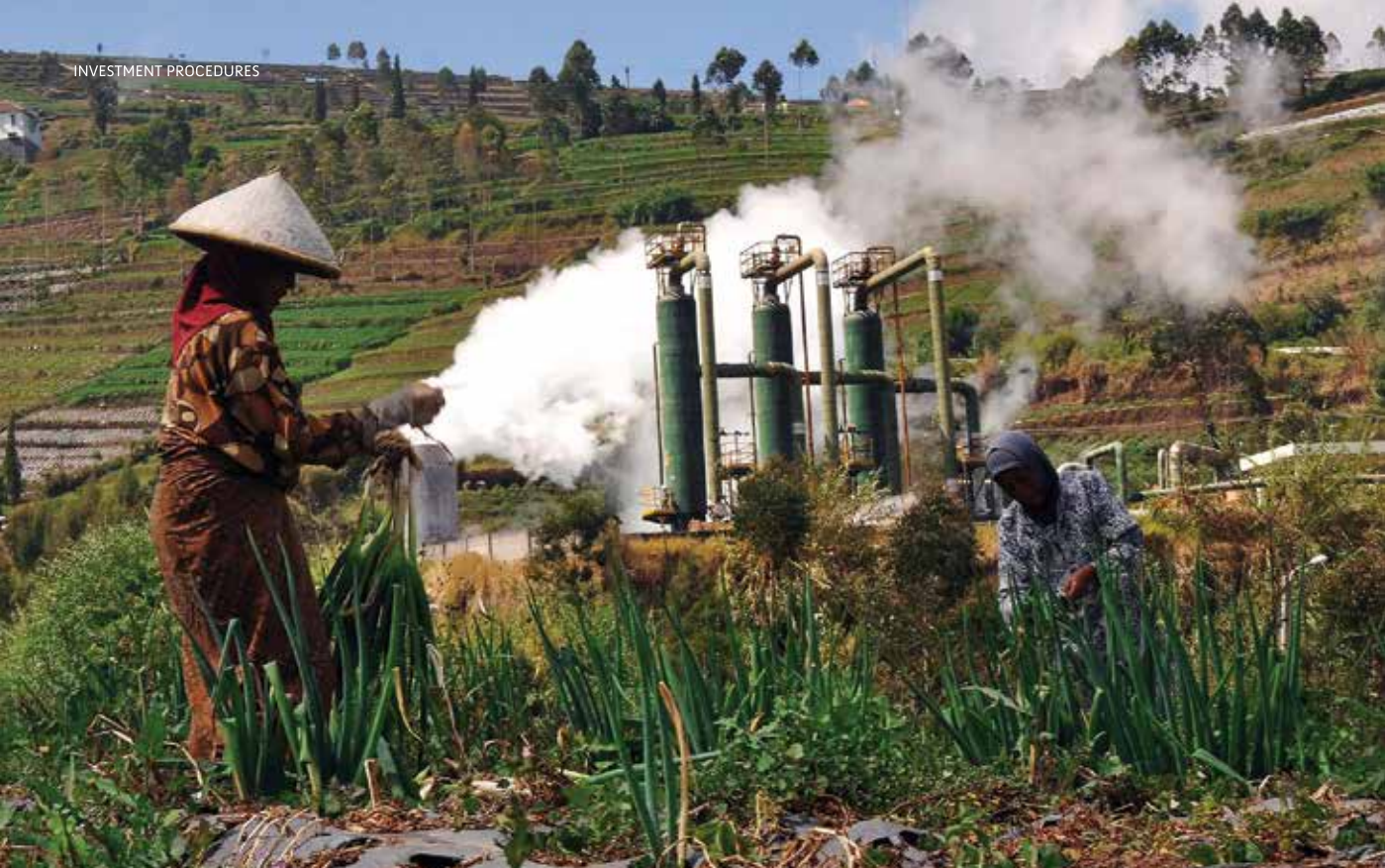
Photo credit: "Instalasi Sumur Geothermal Dieng", 2016
